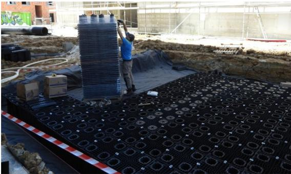
Once the material is available, the pallets of parts must be moved to the excavation with suitable machinery and the Hidrocrates assembled below in the excavation, in this way the movement of materials is minimized. In large tanks, it is advisable to distribute the material in such a way as to minimize movement. Before placing the first block it's advisable to plan the mounting assuring that it respects the alignment and distances of the
