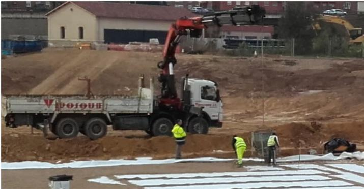
In upper water inlet tanks by infiltration, it is convenient to insert a sheet of geotextile layer over all the surface of the tank to allow that the clogging it's located on it, and if it's necessary to replace it's only necessary to change this geotextile sheet.
