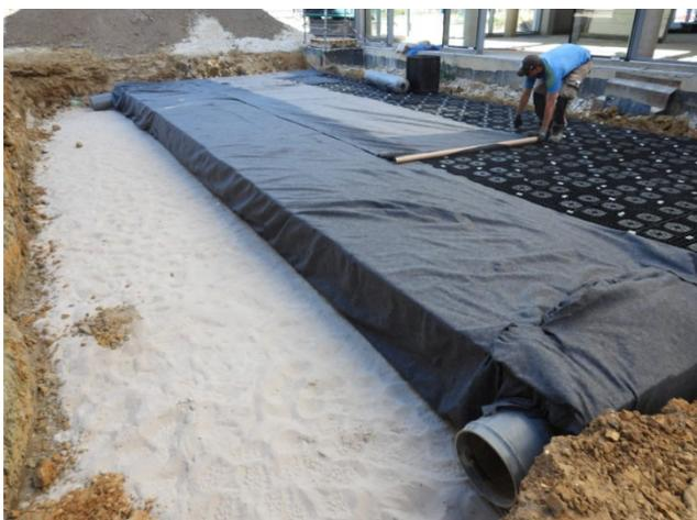
Once finished the deposit, proceed to cover it with the geotextile, mark where the inlet and outlet holes are, the coupling piece for the inspection boxes or the holes for the ventilation stacks.
