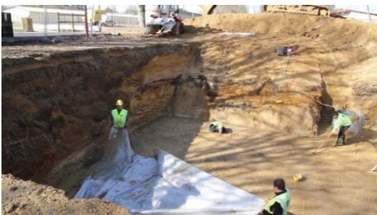
The structure must be completely enclosed with a suitable geotextile, cut out the different sheets on the way that they cover the entire surface and have the enough length to enclose the entire structure. When it is spreading out over the base, if you need some sheets, it's necessary to overlap them at least 30 cm, and avoid the formation of creases.
