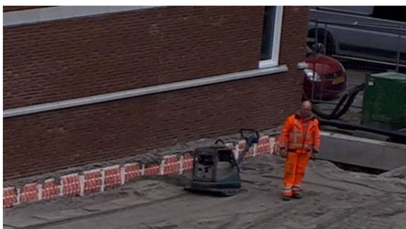
Start with the peripheral filling on the four sides and tiers of 40 cm, before the next tier filling proceed to compaction, will be used a flat compaction unit until compacting greater than or equal to 98% of the proctor modified.
